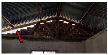
Close open areas between walls and roof with bricks and plaster.
