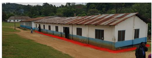
• Dig a 50 cm wide and 20—30 cm deep ditch around the building and fill in the demolition waste. At the end add small stones on top
